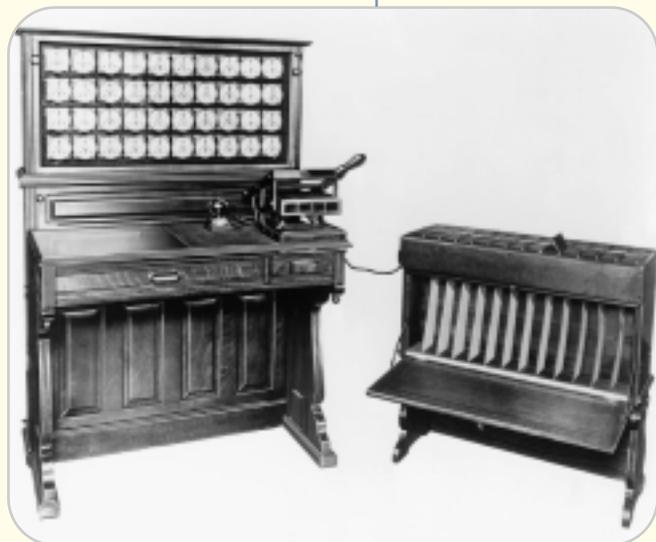
**Mark I** (1943) In a partnership with Harvard University, IBM creates a huge, programmable electronic calculator that used electromechanical relays as switching devices.
